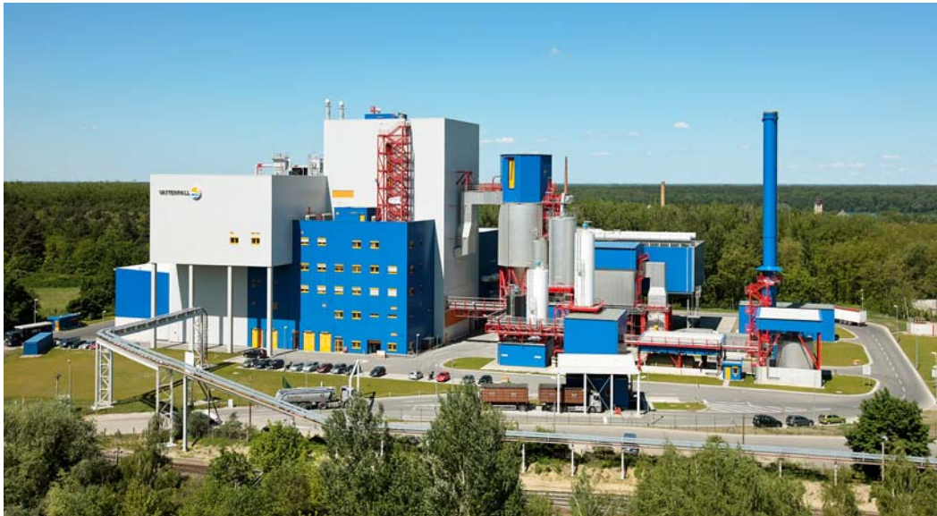
Picture/Graph 5: Waste and biomass to energy plant IKW Rüdersdorf
